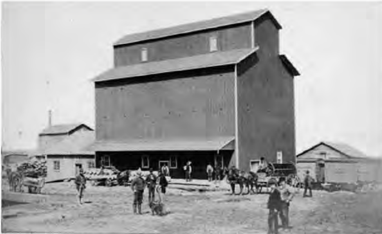
Currie's Grain Elevator (1877) Source: Scugog Shores Museum
