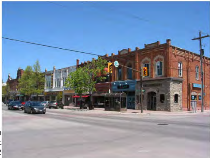
Collingwood Downtown Heritage Conservation District Est. 2002
