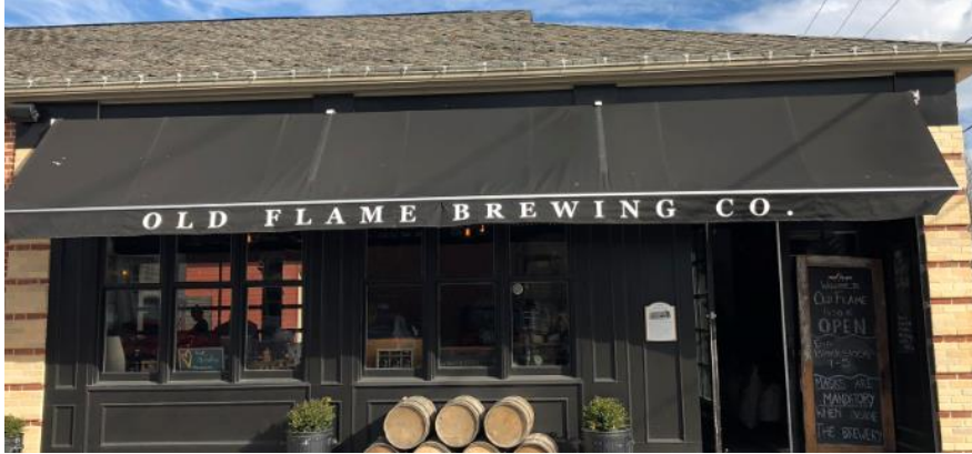
Retractable awning with business name on valance.
