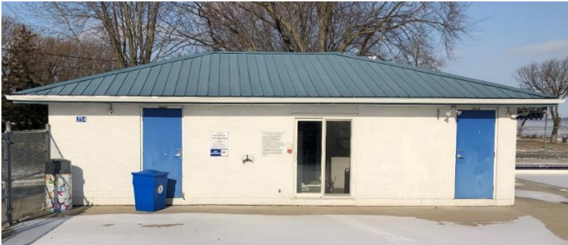
Existing Changeroom Building
